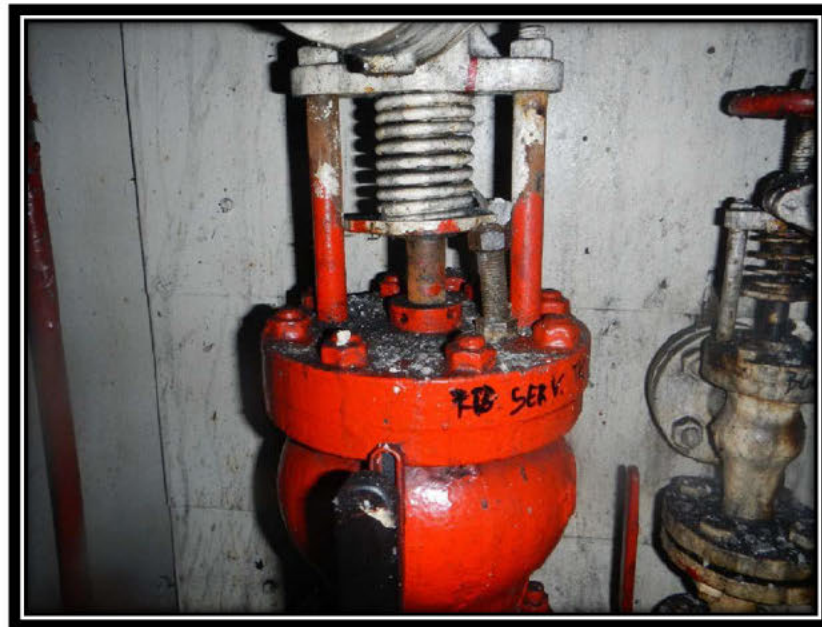
Figure 20; Post Casualty photo of Fuel Oil Service tank blocked open with bolt.
